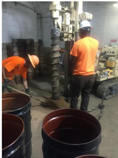
*Installation of electrode to be used for Electrical Resistance Heating.*
