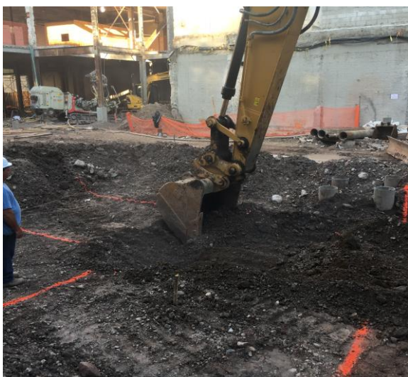
View of hot spot excavation on Site.
