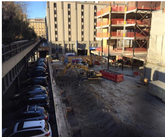
Overview of the Site facing south towards 21 st Street.
