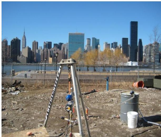
*View of a typical injection well installed at Parcel 8.*
